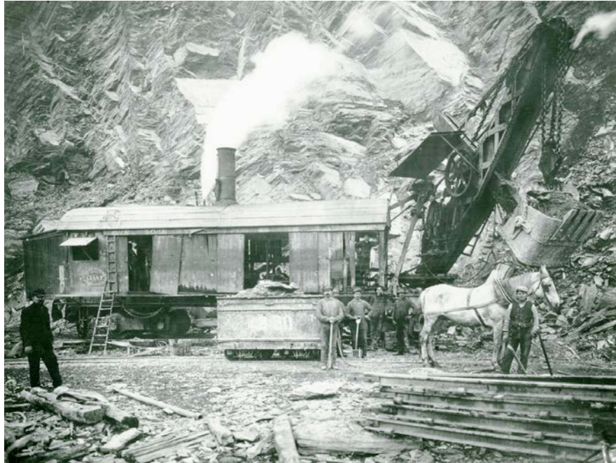
Elmhurst-Chicago Stone Company's first steam shovel, c. 1915. M2014.1.704
